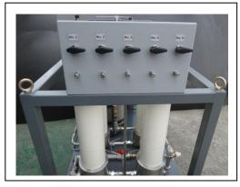
Sample line with isolate valve, for purity analyzing at each section.
