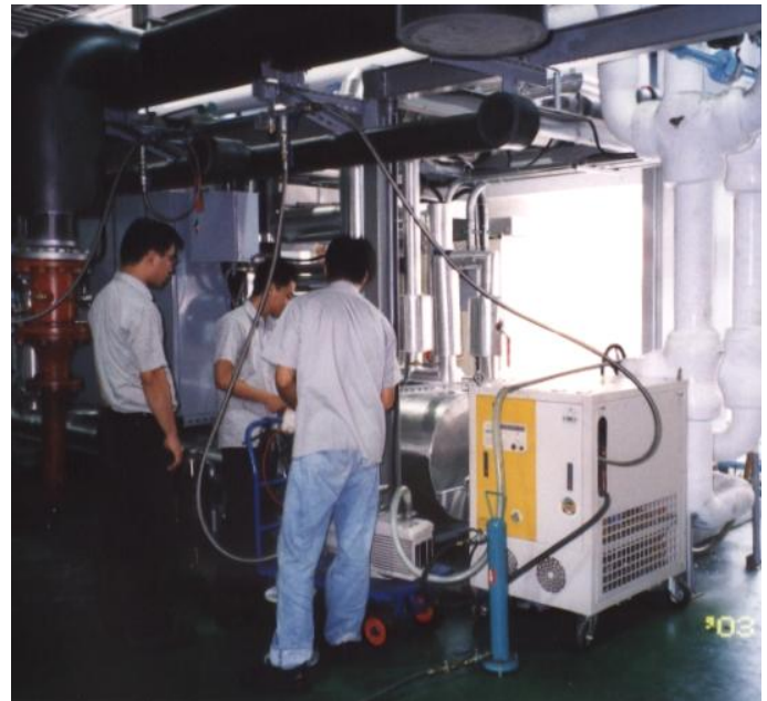
Recovery and Recycling Refrigerant at Compressor Efficiency Testing station.
